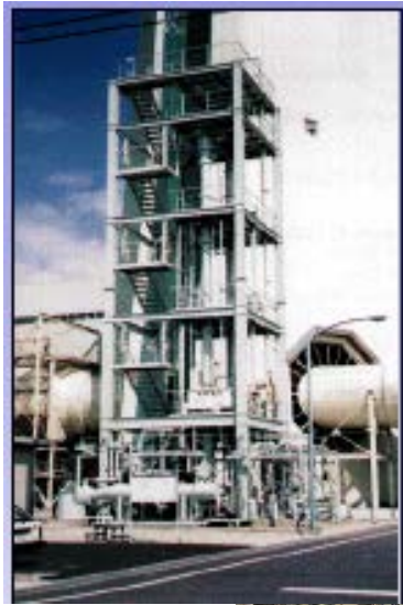
Nanko Pilot Plant (2t/d)
