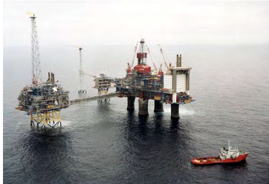
Sleipner, deep saline aquifer, Norway, 1 Mt CO 2 /y since 1996
