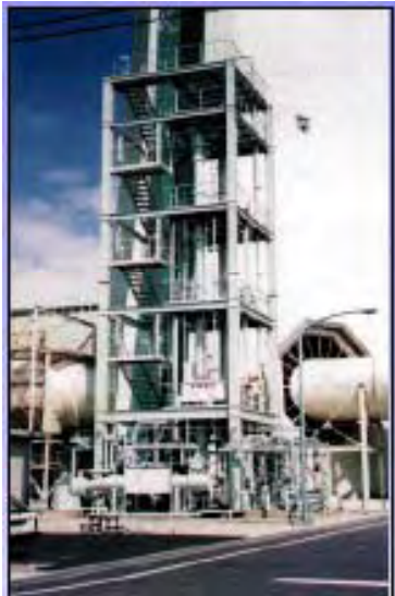
Nanko Pilot Plant (2t/d)
