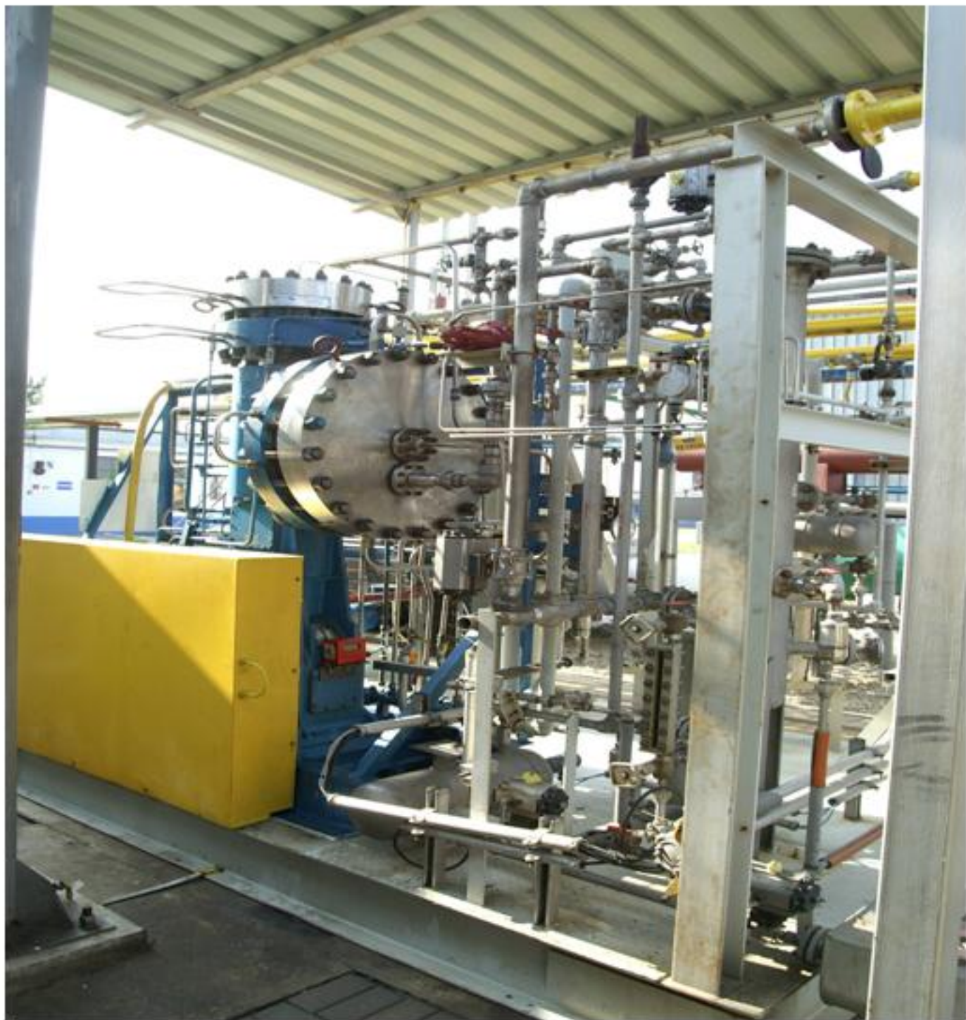
The view of 2-stage diaphragm compressor
